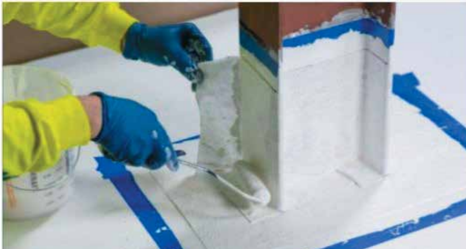
Figure 5. Application of standard liquid-applied flashing on an I-beam.
